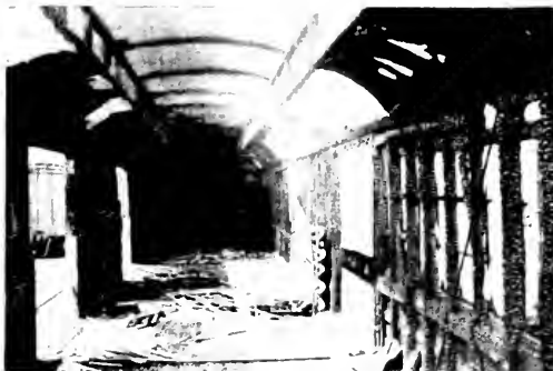
Interior of Wooden Car after Fire.
